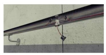
After completing the electrical connection, the plastic installation housing is inserted. The luminaires are mounted flush with the handrail. To explain this installation, there is a video on our website www.meyer-lighting.com.
